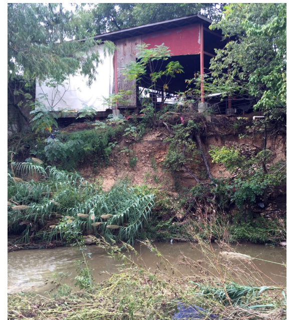
Severe erosion threatens resources along lower Waller Creek.
