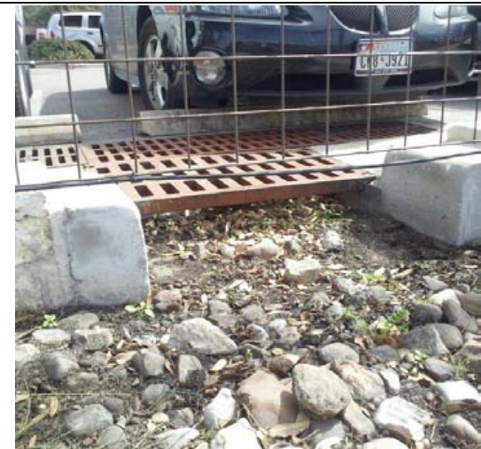
Figure 15 - Clogged inlet (COA, n.d. Green Stormwater Infrastructure Maintenance Manual )
