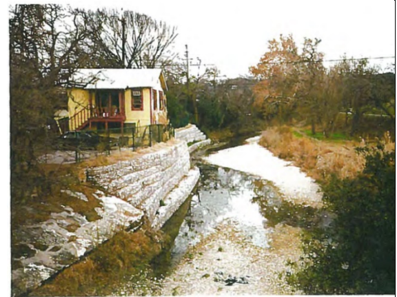
Figure 28 - New gabion along west bank looking upstream from 10th St. Bridge, 1997 (Hegemier, T., 2016)
