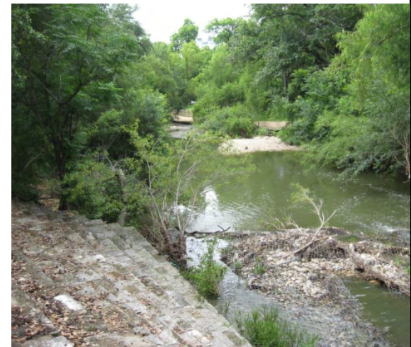
Figure 27 - Damaged gabion mattress, downstream of 9th St., Shoal Creek (Hegemier, T., 2016)
