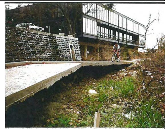
Figure 26 - Cribwall above washout behind hike & bike trail upstream of 6th St. Bridge, looking downstream, 1997. (Hegemier, T. 2016))
