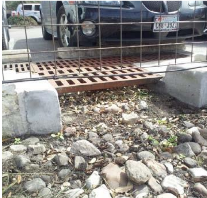
Figure 14 - Clogged inlet (COA, n.d. Green Stormwater Infrastructure Maintenance Manual)
