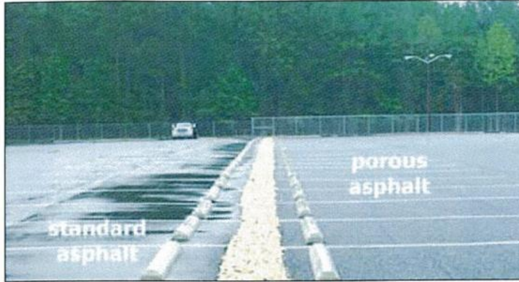
Figure 15 - Porous pavement (BRWM, n.d.)
