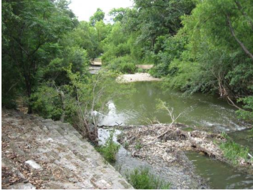
Figure 24 - Damaged gabion mattress, downstream of 9th St., Shoal Creek (Hegemier, T., 2016)
