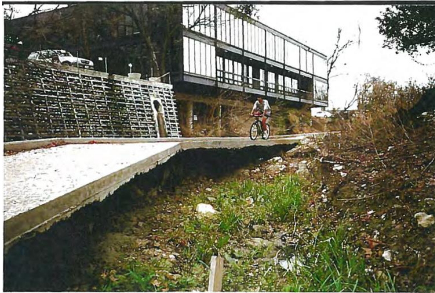
Figure 26 - Cribwall above washout behind hike & bike trail upstream of 6th St. Bridge, looking downstream, 1997. (Hegemier, T. 2016)
