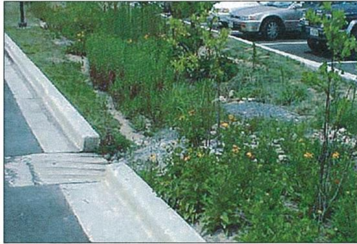
Figure 19 - Bio-Swales (BRWM, n.d.)
