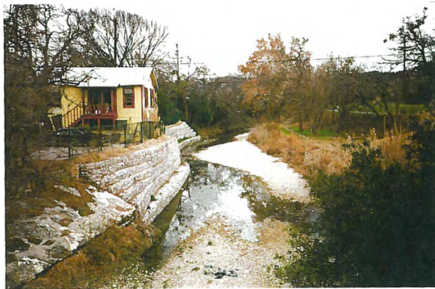
Figure 25 - New gabion along west bank looking upstream from 10th St. Bridge, Shoal Creek, 1997 (Hegemier, T.)
